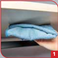
1 Clean grease and dust carefully from the surface for better adhesion
